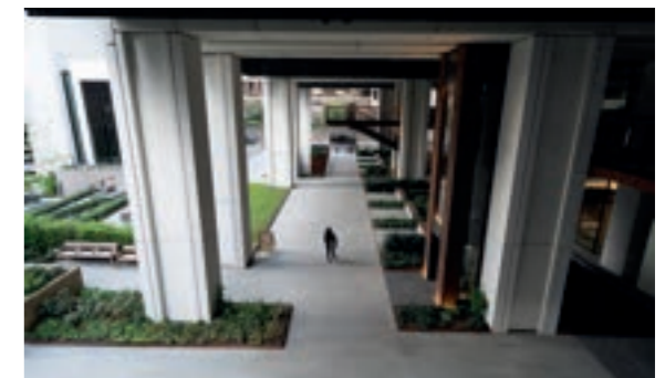
The existing footings and columns of Norco House could be revealed, creating a flowing connection between building and external space
