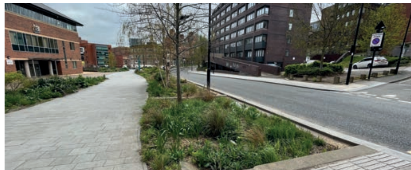
Rain gardens planted between the carriageway and footways soften the streetscape
